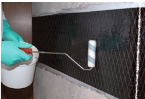
Application of MC-DUR 1209
